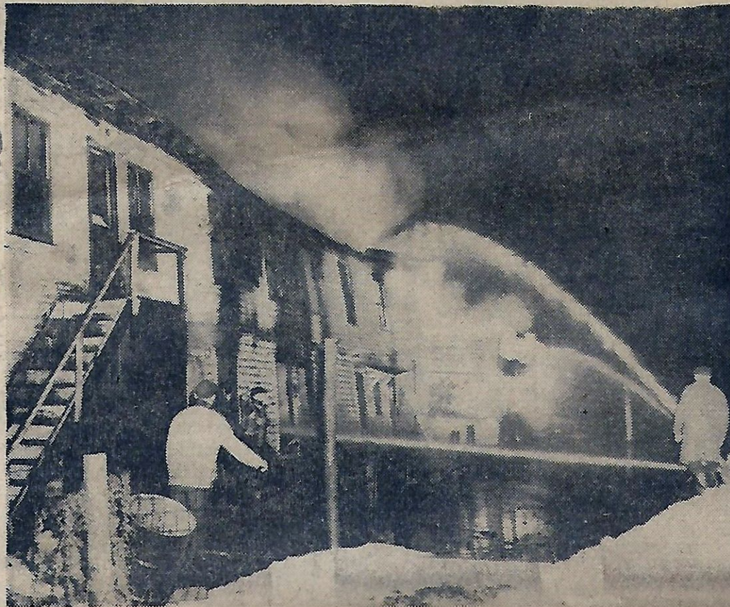
FROM THE BAY —Firemen pump water from Sodus Bay, directly behind the hotel, onto the flames. The early morning fire caused an estimated $40,000 in damages.
